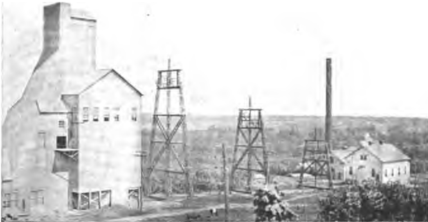
A. SHAFT HOUSE AT BALTIC MINE.
